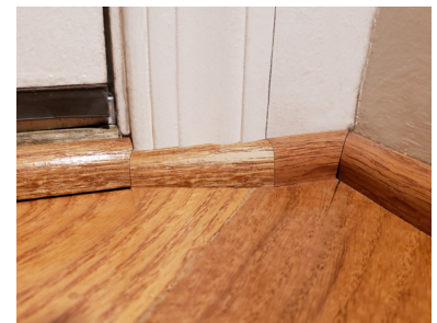
DSM on Exterior doorway
